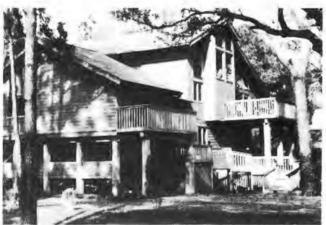
Figure 4.3. Elevation by Posts
