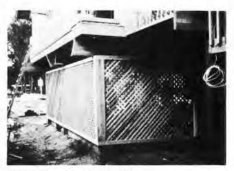
Figure 4.54. Breakaway Walls
