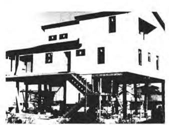
Figure 4.14. Pile Foundations
