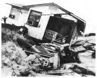
Figure 2.3. Erosion Caused This Foundation to Collapse.
