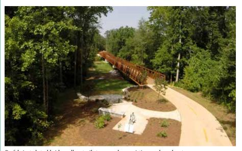
Prefabricated steel bridges allow trails to cross above existing roads and waterways.
