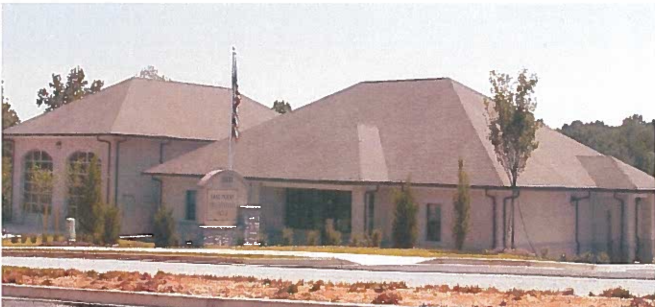
Fire Station No. 3, Located at 3800 North Commerce Drive Built in 2006
