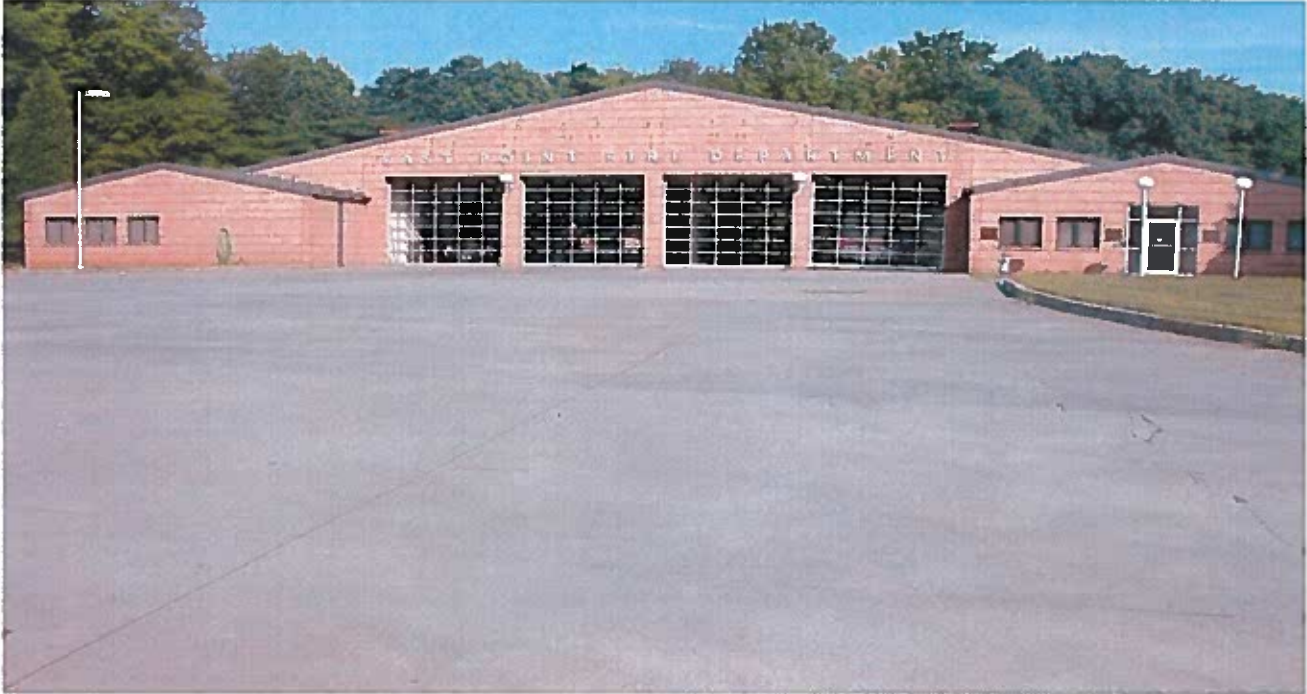
Fire Station No. 2, Located at 3171 Norman Berry Drive Built in 1994
